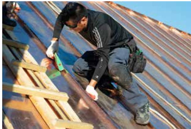
Finishing the seams on Woodend's third floor copper roof.
