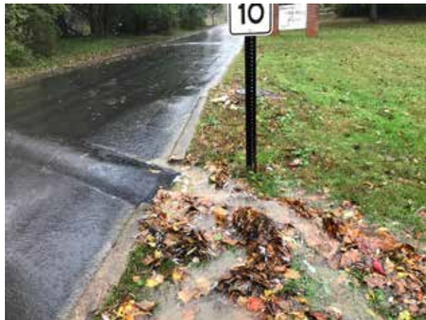
Woodend's new speed bumps divert water from the driveway to the meadow.
